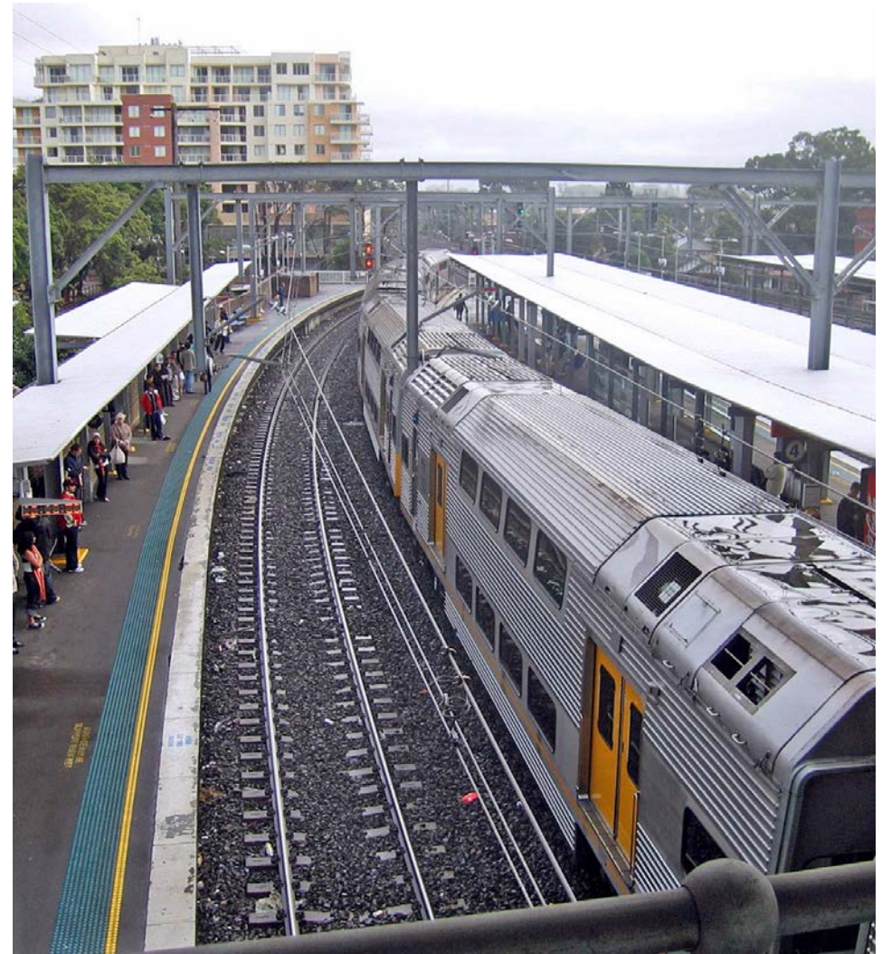
Source: Flickr Images, Ashfield Station
